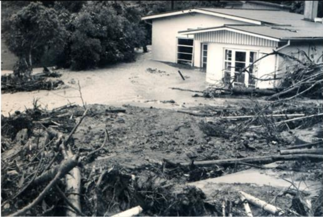
51 Elmslie Rd, Pinehaven (Storm on 20 December 1976)
