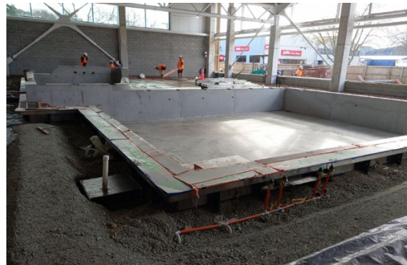
Junior leisure pool slab foundation
