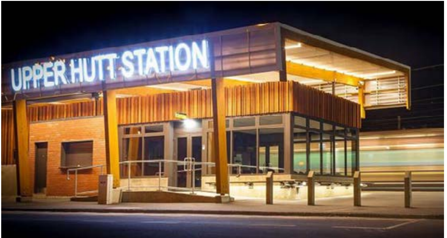
Picture: Upper Hutt Railway Station
