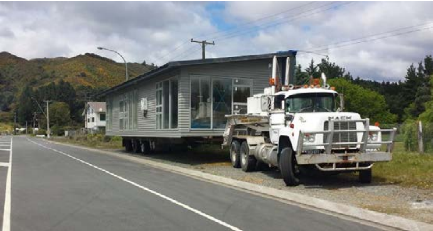
Picture: Matrix Homes module on trailer from factory, matrixhomes.co.nz
