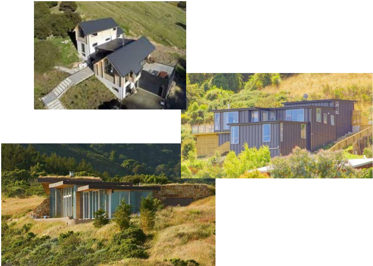
Figure 15 Examples of different building typologies that could be used on Eastern and Southern Hills. These buildings are designed to sit in the landscape either as a small platform building or a collection of building forms with a similar material composition down or up a slope. Use of dark roofs and
