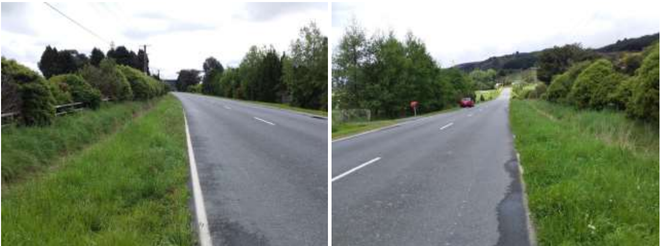
Photos 1 & 2: Mangaroa Valley Road from Site Frontage
