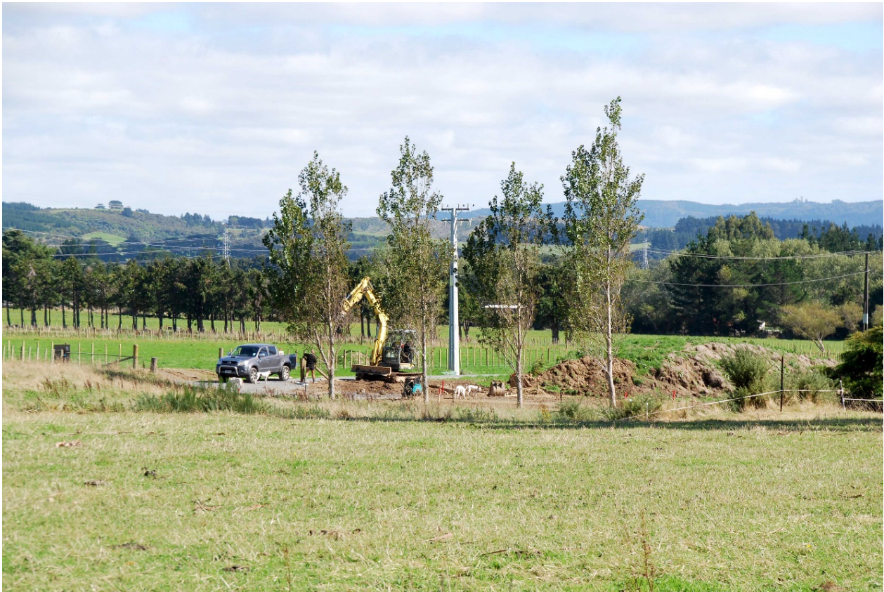
Kaitoke Valley - subdivision development
