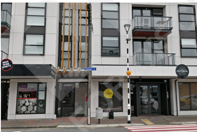
PHOTO 12 - DIFFERENCE IN ENTRANCE DESIGN BETWEEN RESIDENTIAL AND COMMERCIAL ACTIVITIES (PETONE, LOWER HUTT)
