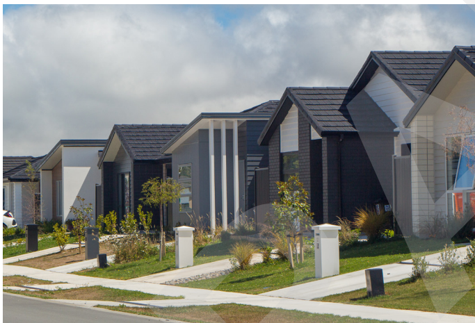
PHOTO 9 - BREAK UP OF MASS THROUGH FAÇADE AND ROOF ARTICULATION (WALLACEVILLE, UPPER HUTT)
