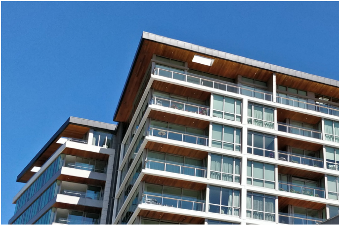
PHOTO 10 - ROOF FORM INTEGRATED WITHIN THE DESIGN OF THE TOP STOREY
