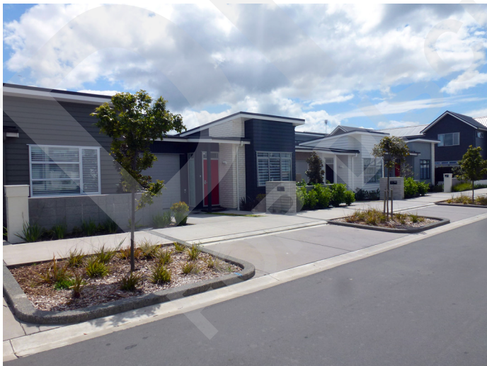
PHOTO 13 - CONSISTENT PATTERN OF GARAGES WITHOUT DISRUPTING PEDESTRIAN MOVEMENT ALONG THE FOOTPATH (HOBSONVILLE, AUCKLAND)
