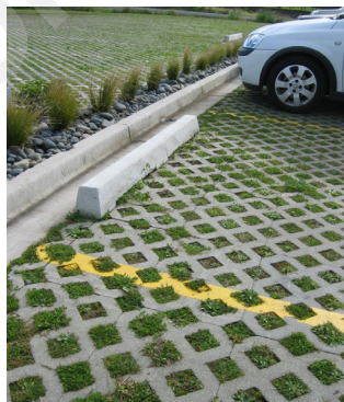
PHOTO 7 - PERMEABLE PAVING (WELLINGTON)
