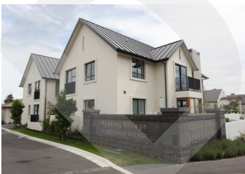
Multi unit dwelling / apartment
