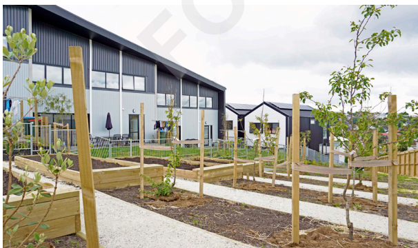
PHOTO 3 - COMMUNAL OUTDOOR SPACE (KUPE STREET HOUSES, AUCKLAND)
