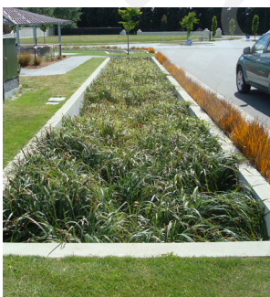
PHOTO 5 - RAIN GARDEN (ROLLESTON)
