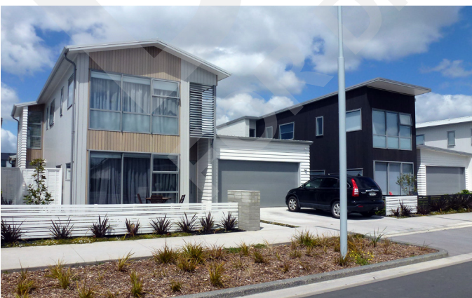
PHOTO 13 - VARIATION IN COLOUR, ROOF TYPES AND MATERIALS (HOBSONVILLE, AUCKLAND)
