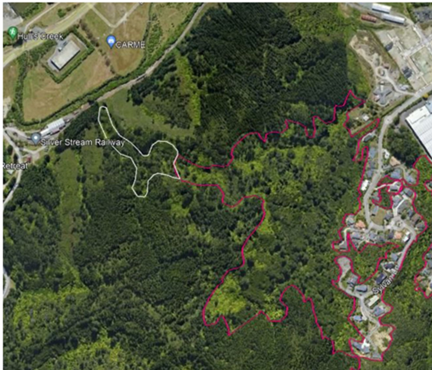
Figure 3 – Combined extent of SNA for the Silverstream Spur with magenta outline showing extent of significant indigenous vegetation identified in the 2020 site visit and white outline showing additional extent from 2022 site visit. The combined area, within the Silverstream Spur, is recommended to be identified as the “Silverstream Spur Natural Area” on the planning maps in Appendix 1
