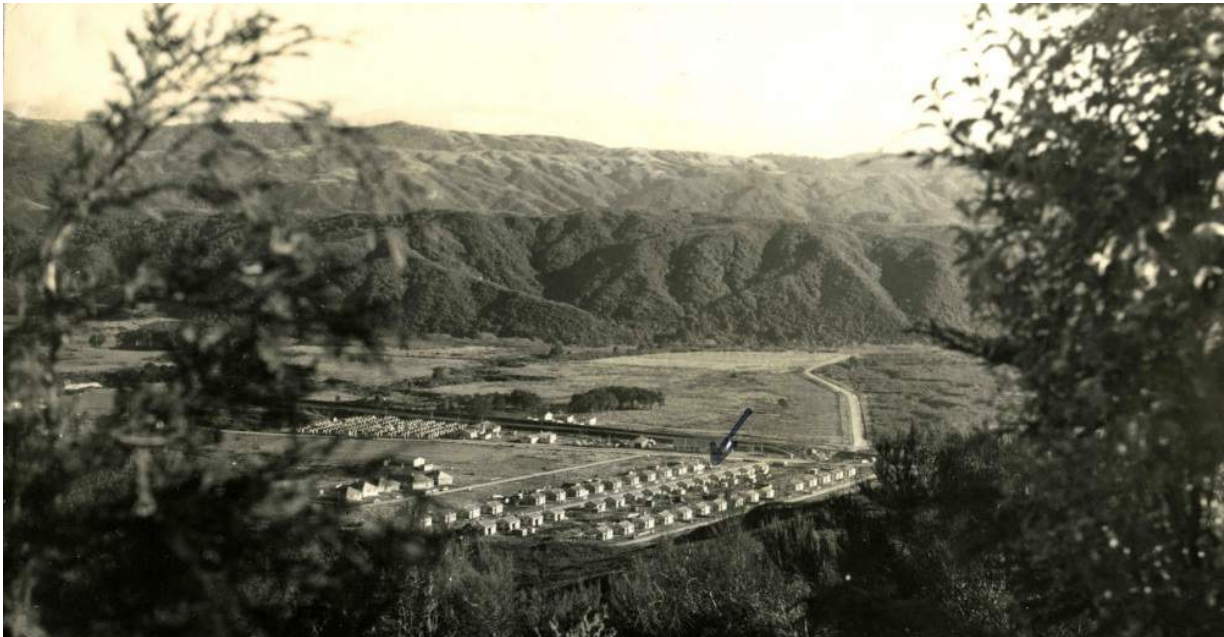
Maymorn tunnel camp 1952. Image source: Upper Hutt Library
