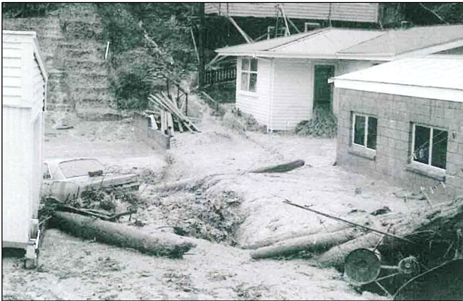
Figure 5. Flooding at 47 Elmslie Road during the 1976 flood 11
