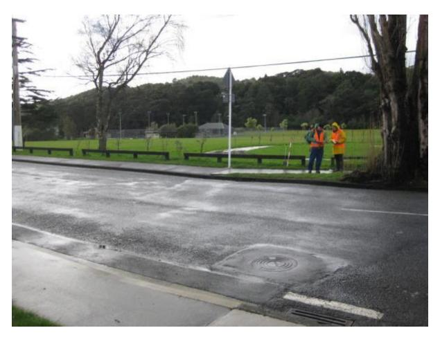
Fig. 20. Secondary overflow channel over Whitemans Road with possible minor earthworks required on Pinehaven Reserve. This upper part of the reserve area is artificially levelled.
