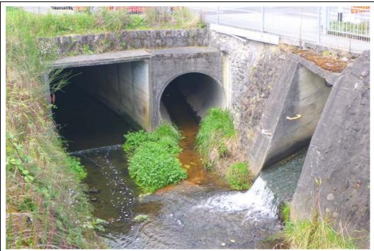
The confluence of Pinehaven Stream with Hull Creek. The left-hand box culvert is the outlet of a piped section of Hull Creek, the middle circular pipe is the outlet of the Pinehaven Stream flood bypass, and the right-hand outlet is Pinehaven Stream emerging from its lower piped section.
