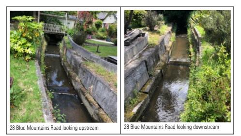
Figure 9 Existing state of Pinehaven Stream channel at 28 Blue Mountains Road showing grade control weirs and concrete block form of banks.
