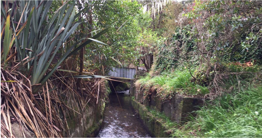
Plate 1: Existing concrete structures in Pinehaven Stream (DCM Urban Design Page 14).
