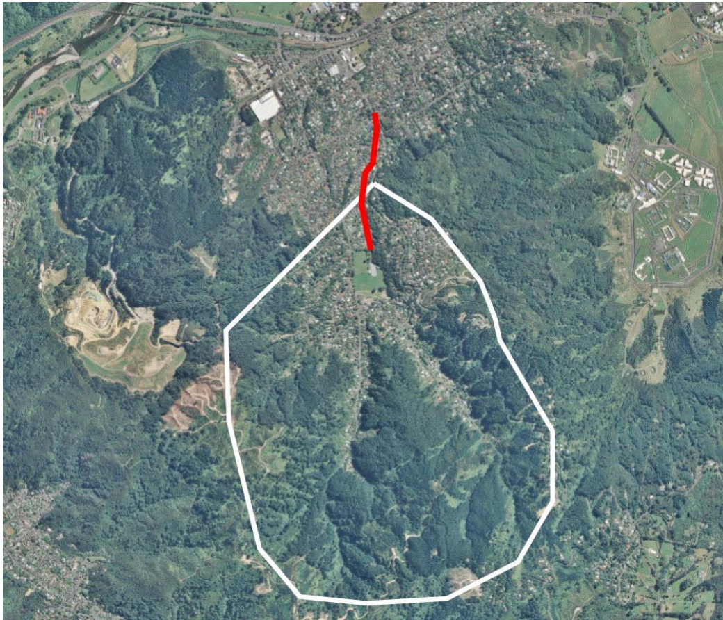
Figure 1: Pinehaven catchment (shown white polyline) and extent of stream upgrade (shown in red line).
