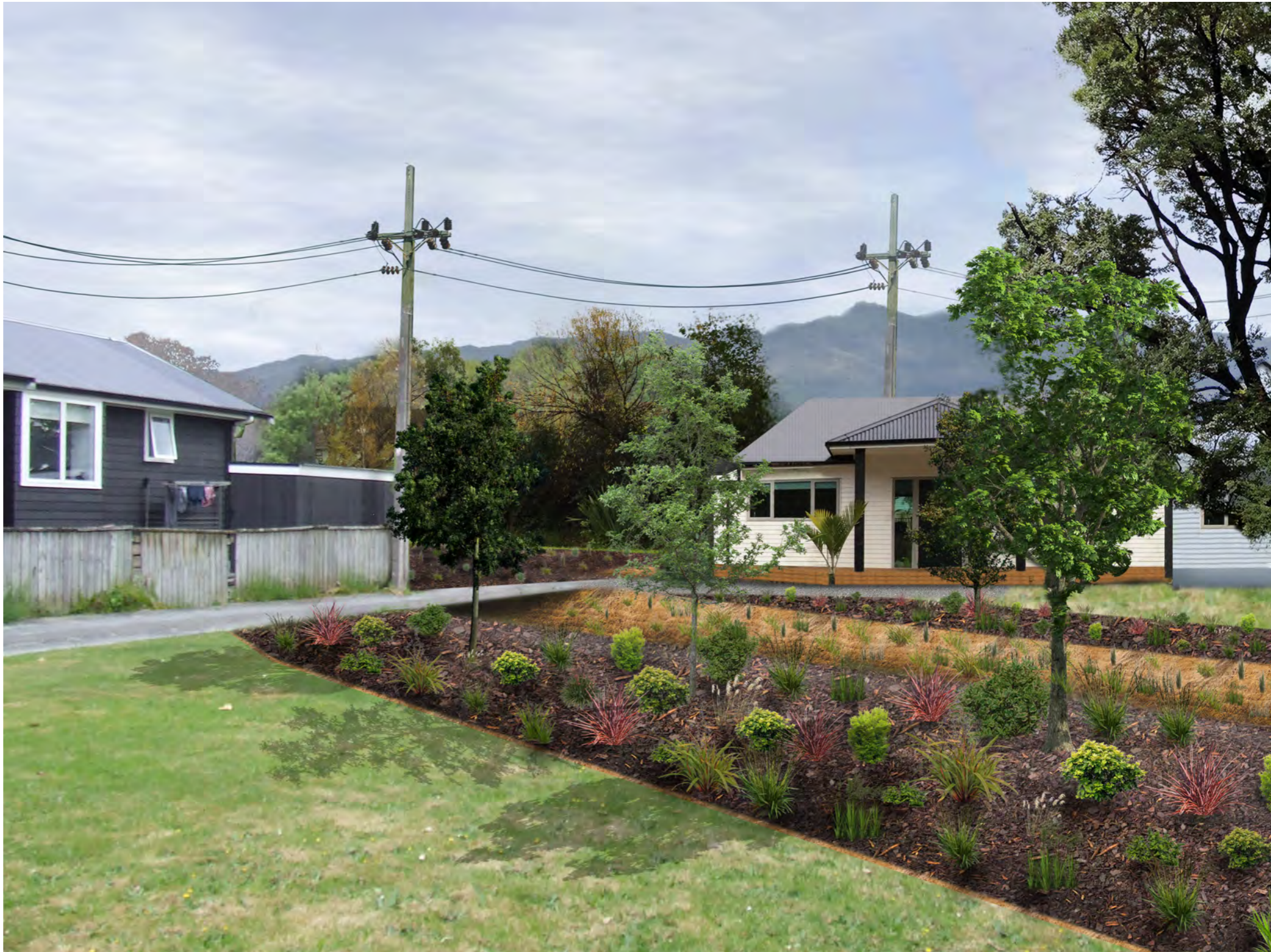
DAY 1 AFTER CONSTRUCTION IS COMPLETED
