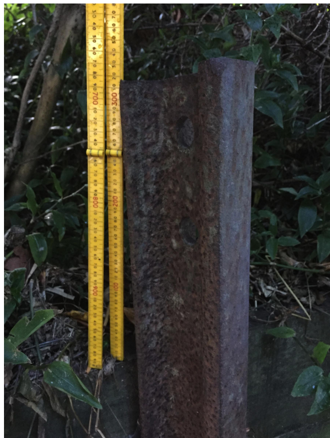
3 - Top of steel post is 317mm above top of retaining wall
