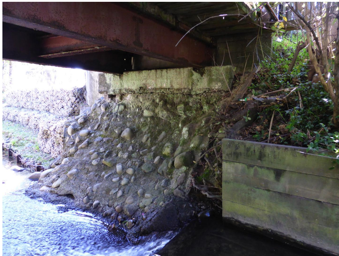
4 - Right Bank at Footbridge
