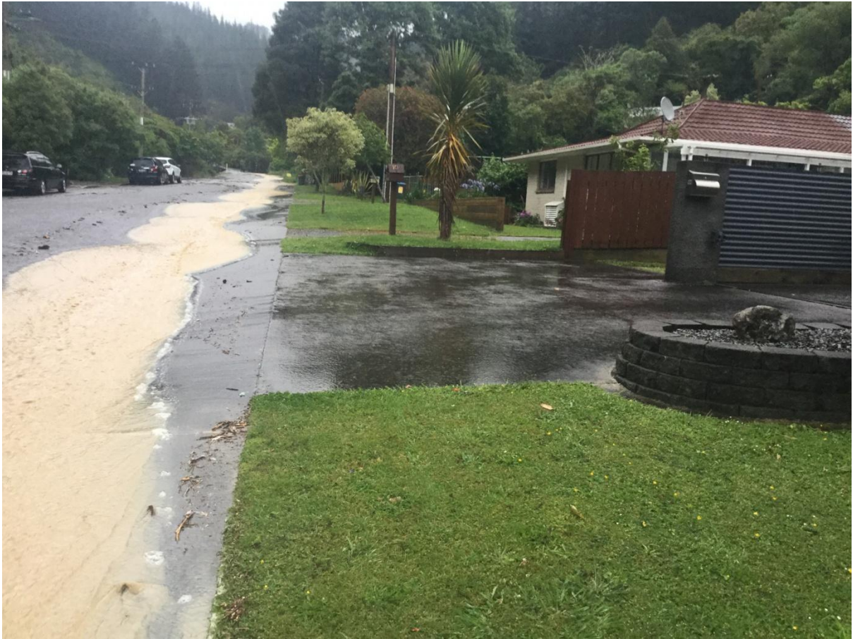
Photograph of secondary flow path caused by undersized culvert and vegetation blocking the channel below the culvert at 122 Pinehaven Road.
