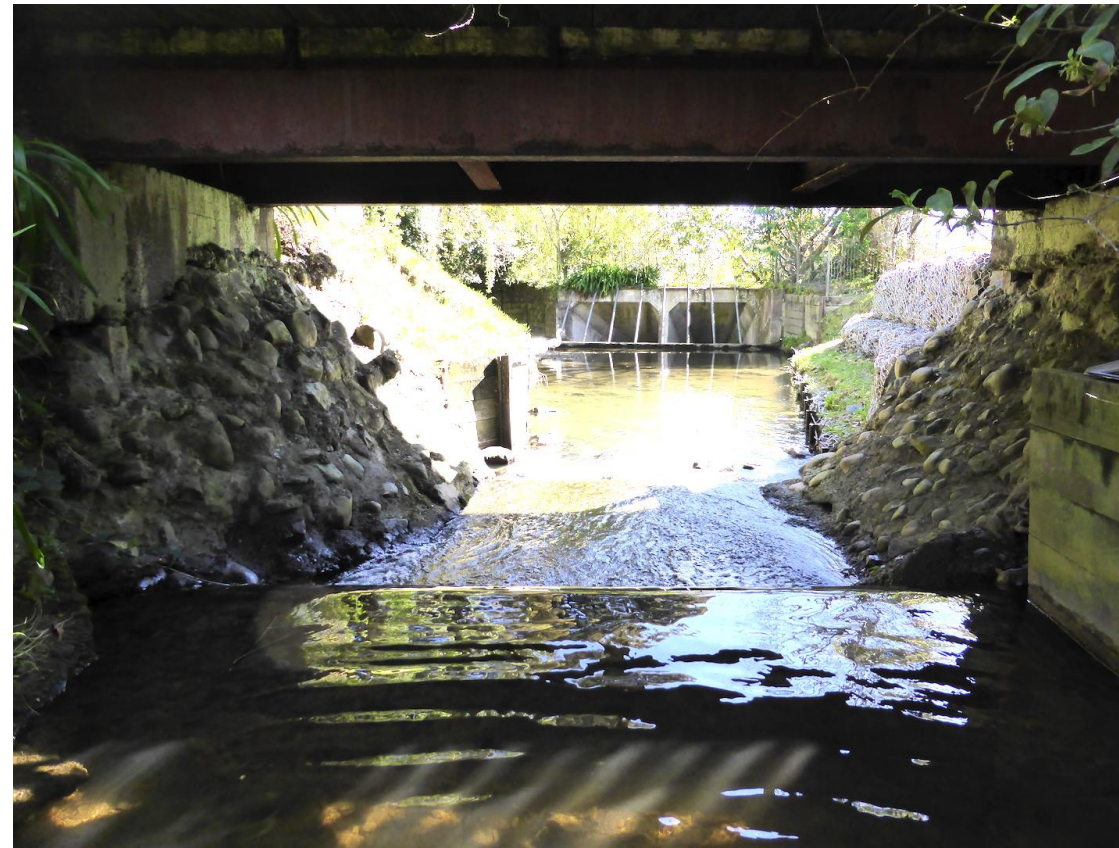
2 - Weir under Footbridge
