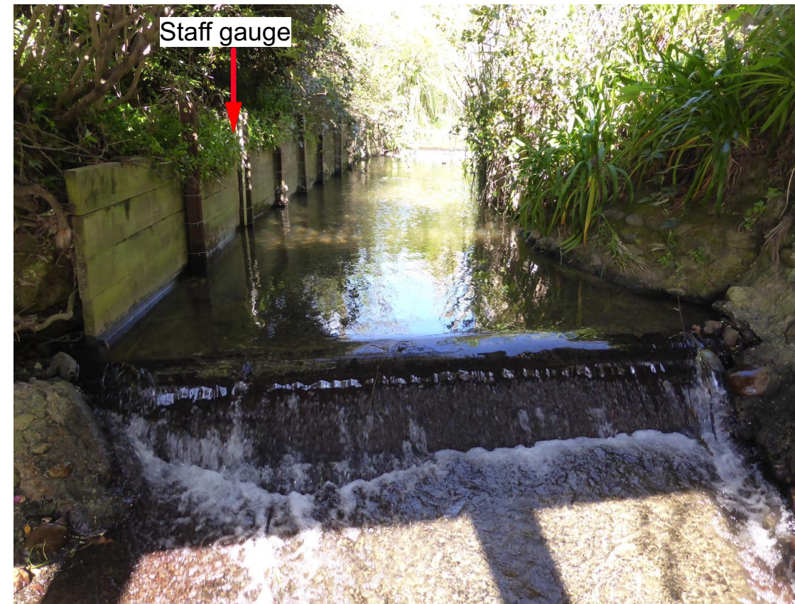
5 - Under footbridge (looking upstream at weir)
