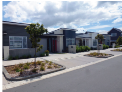
PHOTO 12 - CONSISTENT PATTERN OF GARAGES WITHOUT DISRUPTING PEDESTRIAN MOVEMENT ALONG THE FOOTPATH (HOBSONVILLE, AUCKLAND)
