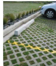
PHOTO 7 - PERMEABLE PAVING (WELLINGTON)
