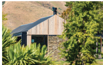
PHOTO 13 - CHOICE OF MATERIALS AS AN INTEGRAL PART OF THE DESIGN (WHITEMANS VALLEY, UPPER HUTT)
