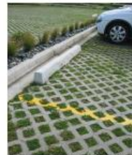
PHOTO 7 - PERMEABLE PAVING (WELLINGTON)
