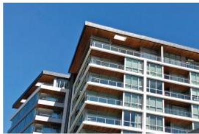
PHOTO 17 - ROOF FORM INTEGRATED WITHIN THE DESIGN OF THE TOP STOREY
