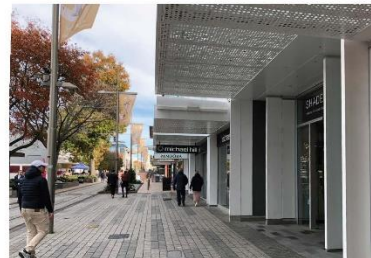
PHOTO 10 - VERANDAHS TO PROVIDE SHELTER, CHRISTCHURCH
