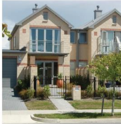
PHOTO 10 - PROVISION OF A CLEAR ENTRANCE AND BALCONY FRONTING THE STREET (NORTHWOOD, CHRISTCHURCH)
