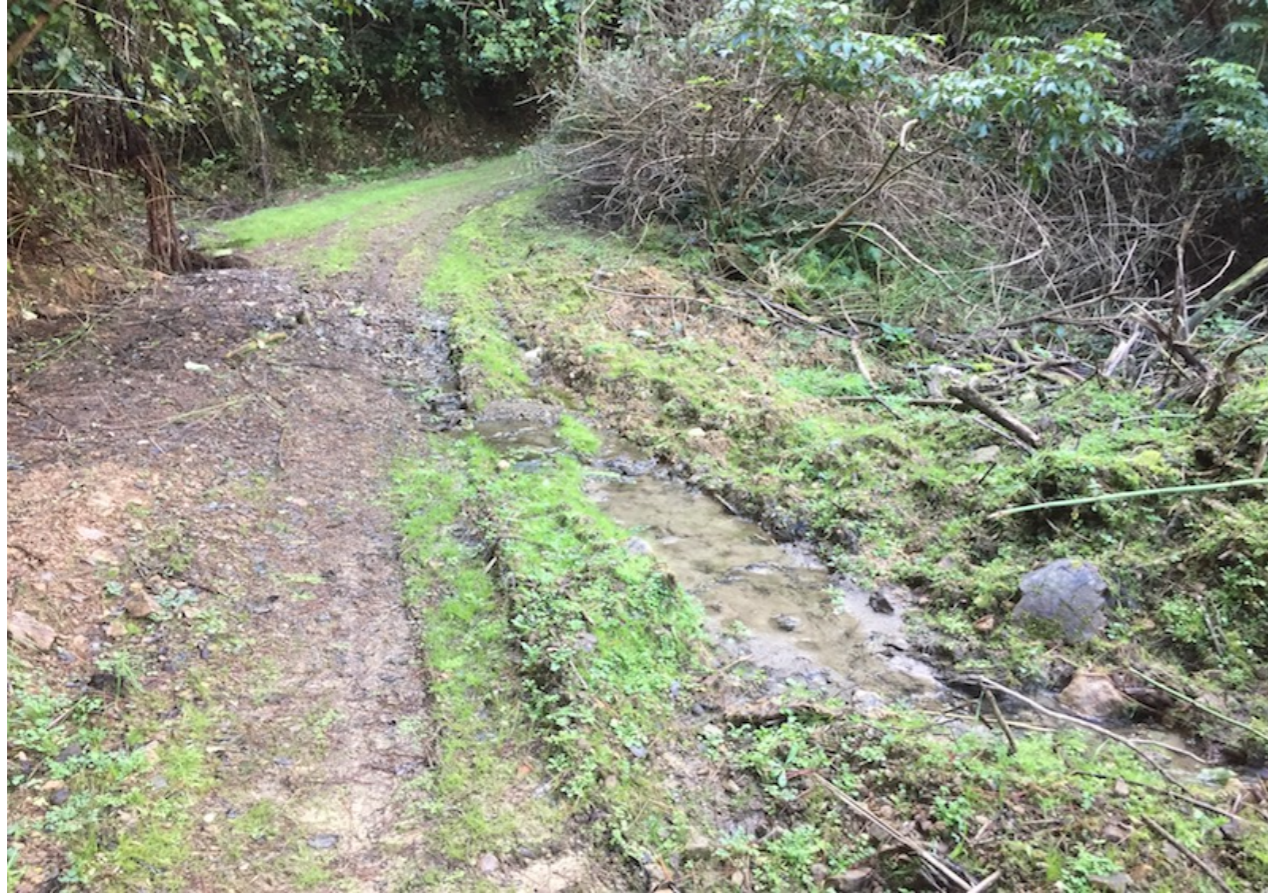
Examples of runoff uphill of the logging road crossing over the road
