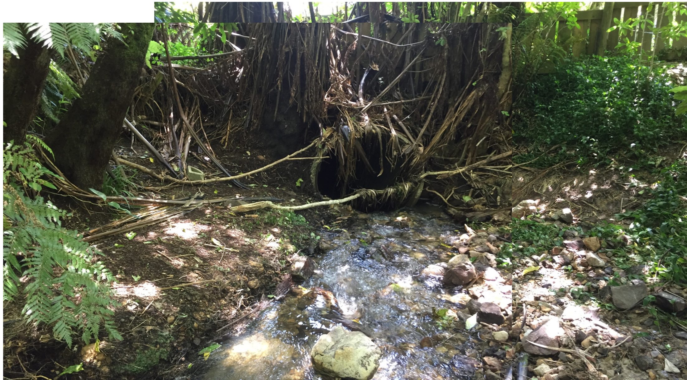
Pinehaven Stream - Sub-catchment B Segment 3 (Contd.): Large open channel flow
