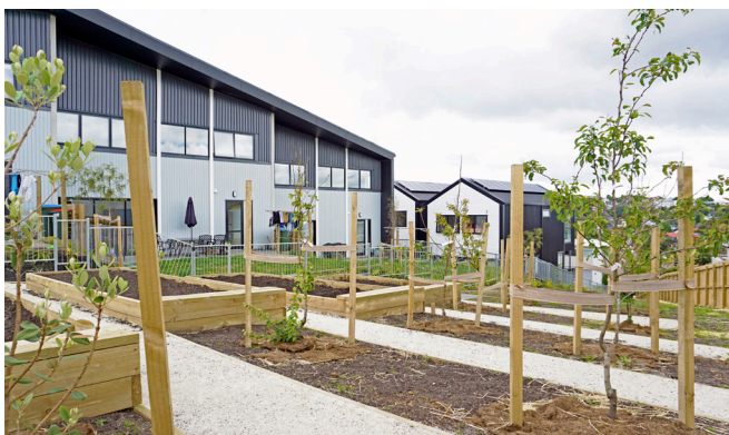
PHOTO 4 - COMMUNAL OUTDOOR SPACE (KUPE STREET HOUSES, AUCKLAND)
