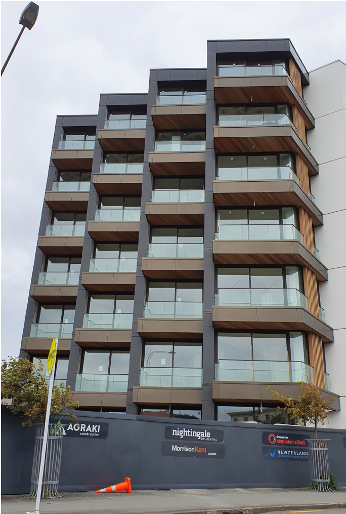
PHOTO 22 - STAGGERED BALCONIES MAXIMISE PRIVACY WHILE RETAINING OUTLOOK AND SUNLIGHT ACCESS (WELLINGTON)
