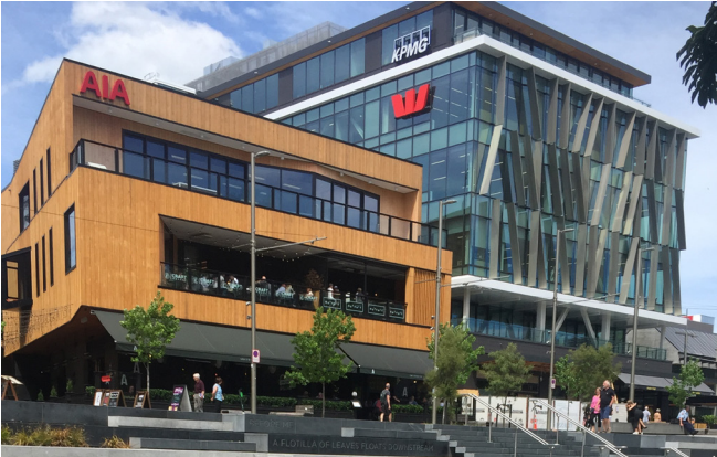
PHOTO 6 - BULK OF THE BUILDINGS BROKEN DOWN BY A BOTTOM, MIDDLE AND TOP, CHRISTCHURCH.
