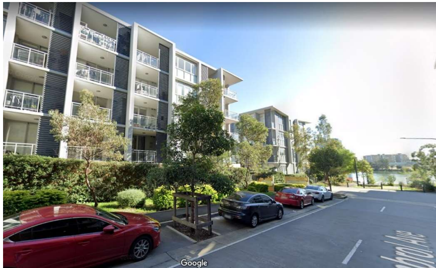
Figure 5 – Timbrol Avenue, Sydney (Google Streetview image)
