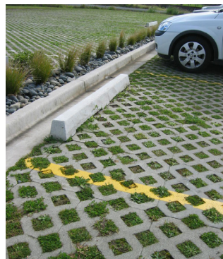
PHOTO 7 - PERMEABLE PAVING (WELLINGTON)
