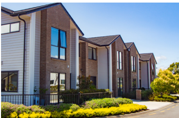
Multi dwelling housing / townhouses
