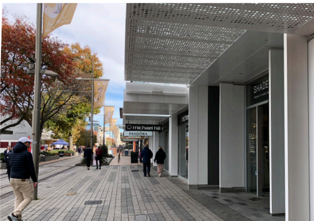
PHOTO 10 - VERANDAHS TO PROVIDE SHELTER, CHRISTCHURCH
