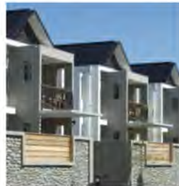
PHOTO 20 - OVERHANGING BALCONIES PROVIDE SHADE IN SUMMER (CLEARWATER GOLD RESORT, CHRISTCHURCH)
