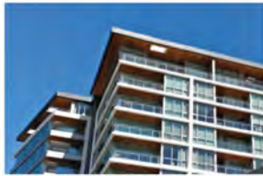
PHOTO 8 - ROOF FORM INTEGRATED WITHIN THE DESIGN OF THE TOP STOREY
