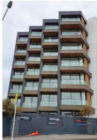
PHOTO 22 - STAGGERED BALCONIES MAXIMISE PRIVACY WHILE RETAINING OUTLOOK AND SUNLIGHT ACCESS (WELLINGTON)
