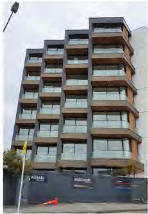
PHOTO 9 – STAGGERED BALCONIES MINIMISE PRIVACY WHILE RETAINING OUTLOOK AND SUNLIGHT ACCESS (WELL HETON)
