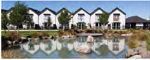
PHOTO 18 - PROVISION OF A RANGE OF BUILDING SIZES AND TYPES CATERING TO A VARIETY OF DIFFERENT LIFESTYLES (DELAMAR, CHRISTCHURCH)
