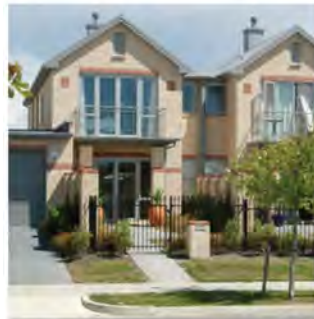
PHOTO 10 - PROVISION OF A CLEAR ENTRANCE AND BALCONY FRONTING THE STREET (GROTHWOOD, CHRISTCHURCH)
