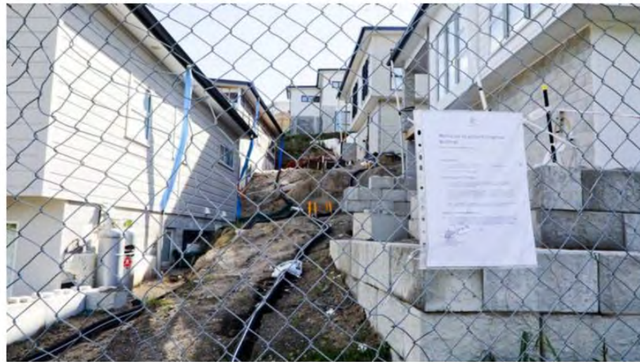
Bella Vista homes in The Lakes subdivision. Photo/file
