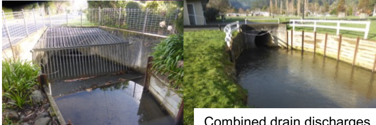
Overflow bypass built in 1980s at 105 Pinehaven Road
