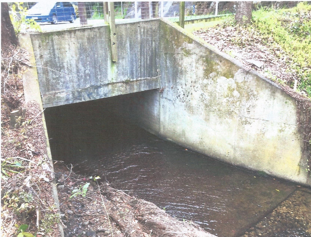
Inlet showing Headwall and wing wall
