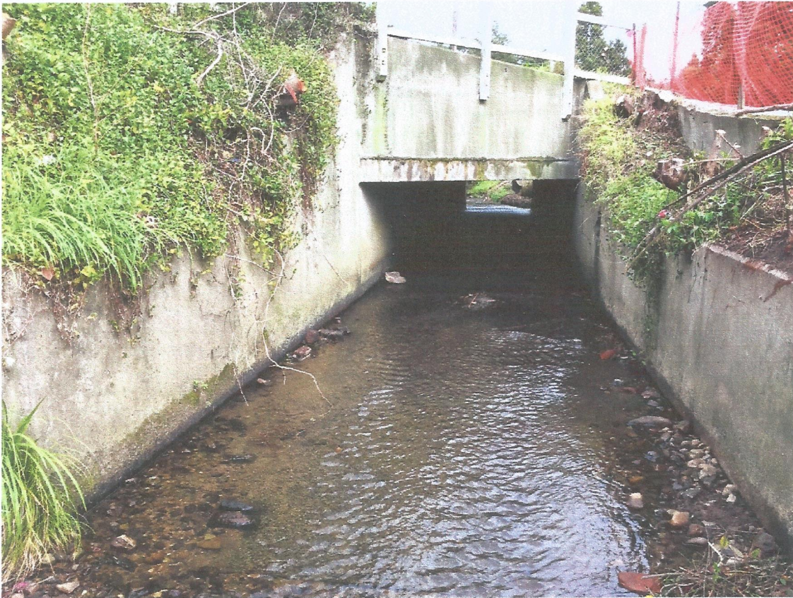
Outlet showing headwall and wing walls
