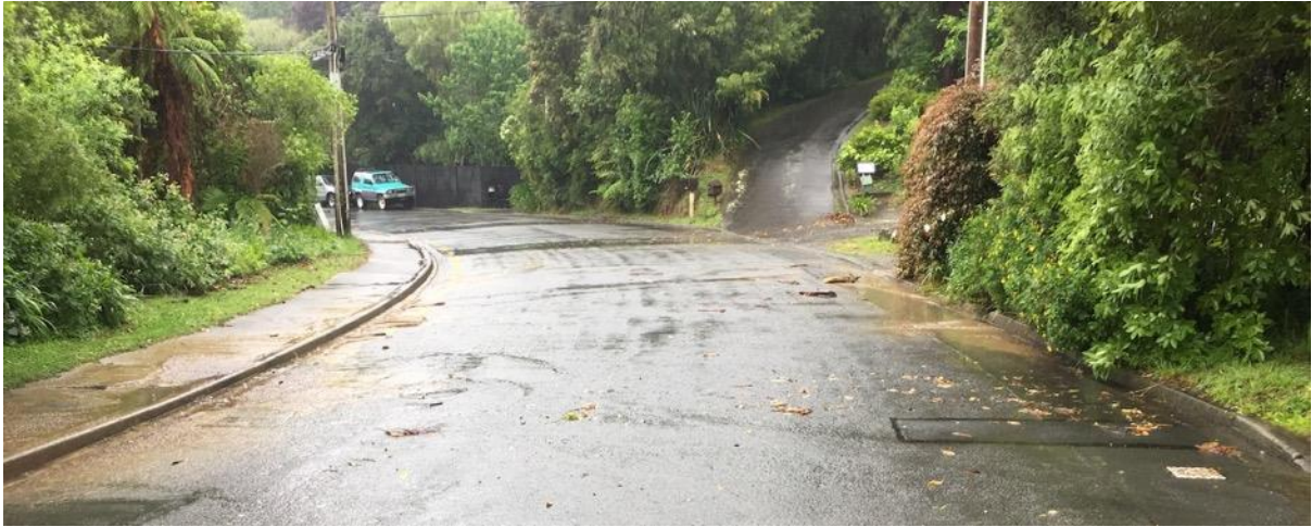
108A Wyndham Rd culvert overtopped
