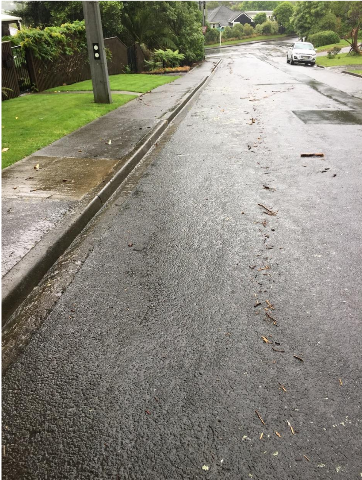
Debris line down Wyndham Rd from overtopped culvert at No. 108A (looking down Wyndham Rd towards Jocelyn Cres.)
