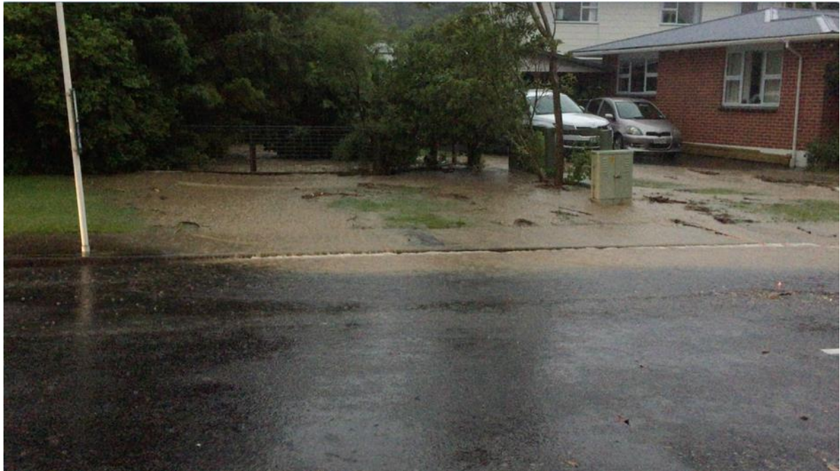
Overtopping of road culvert, adjacent to 4 Sunbrae Drive, 06:21 am
