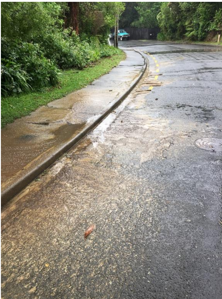
Opposite site of road from overtopped culvert at 108A Wyndham Rd
