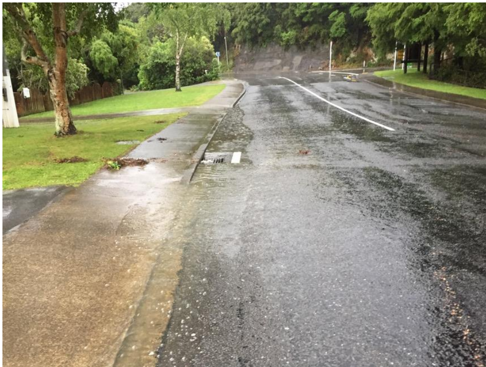
06:56 am – ponding cleared within 5 minutes after sump was unblocked by a resident from No. 2 Pinehaven Road - see resident's statement on next page (p41).
