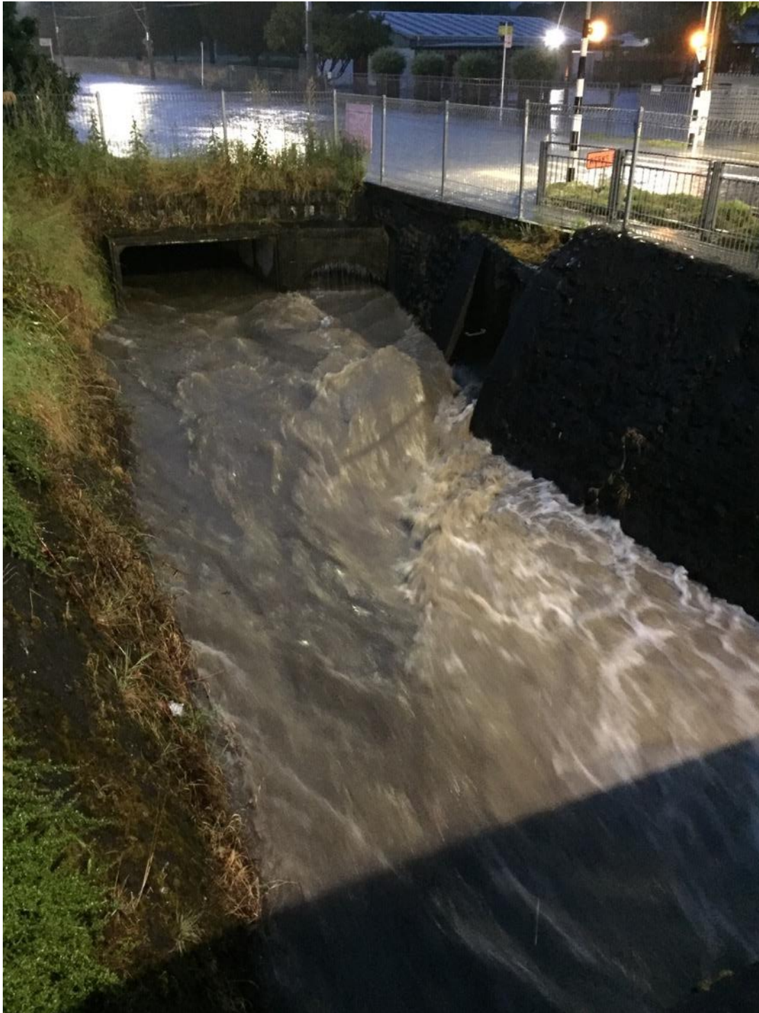
Hulls Creek, discharges from Heretaunga box culvert, Pinehaven bypass and piped stream 05:43 am
